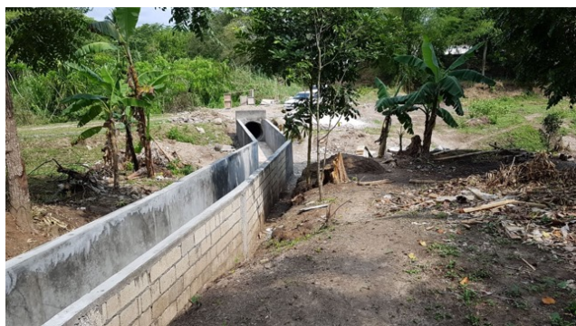
Completed culvert and U drain
