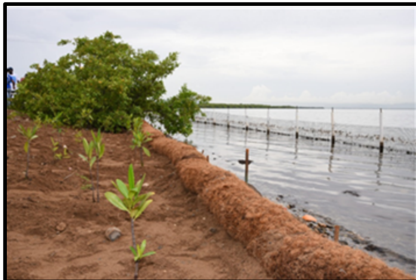
Seedlings planted along the shoreline behind coir logs at Airport Runway
