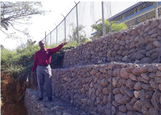
Installed Gabion baskets
