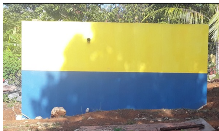
Concrete water storage tank of 20,000 gallon capacity
