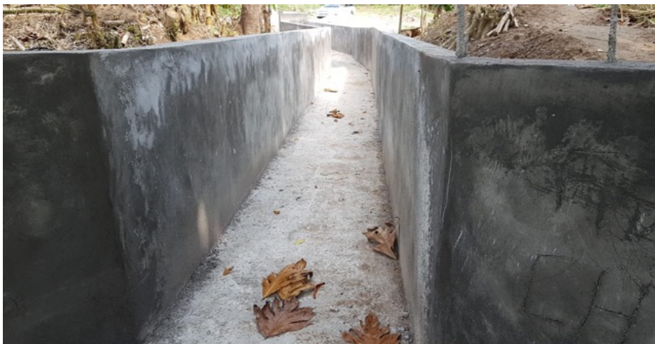
Completed culvert and U drain
