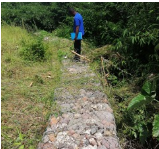
Installed gabion basket
