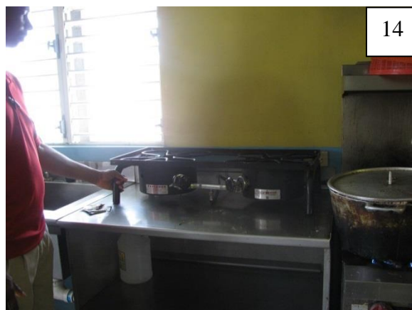
Photo 14 – Stove powered by gas generated from the bio-digester system which is used to prepare meals for the Home. Mr. Whitely demonstrates the process of the gas being generated.
