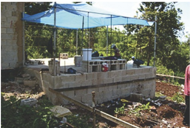
Construction of placement area for water tanks and adjoining abattoir
