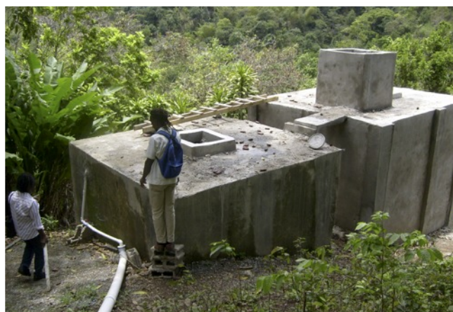
Mount Vernon water storage tanks under construction, with community support and labour
