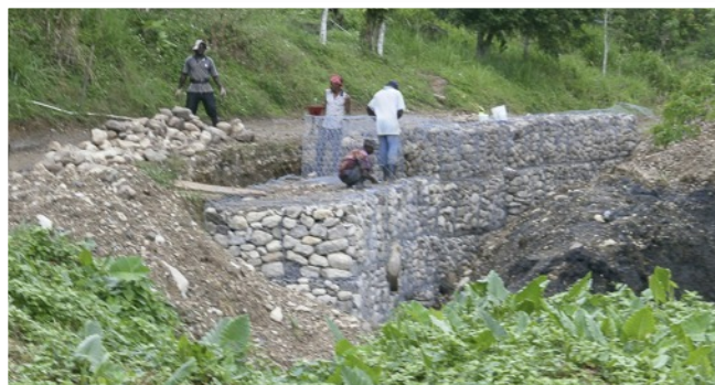
Construction of retaining wall with gabion baskets by the Jeffrey Town Farmers Association in St. Mary, Jamaica
