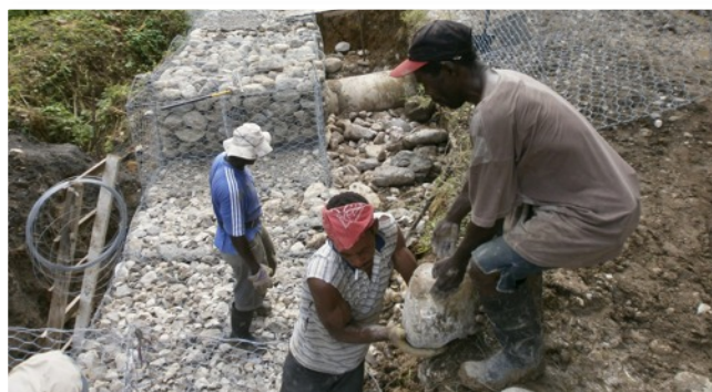
Construction of retaining wall with gabion baskets by the Jeffrey Town Farmers Association in St. Mary, Jamaica
