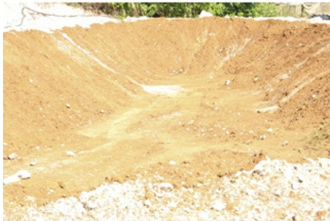
Excavation of land for installation of pond liner
