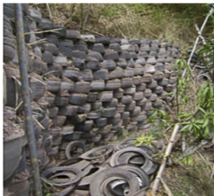
Used tyres being used for hillside stabilisation
