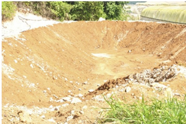
Excavation of land for installation of pond liner
