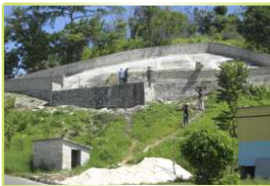
New Works catchment and storage tanks
