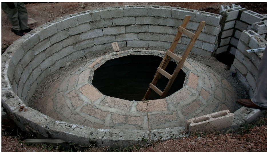
Biodigester under construction at Edwin High School
