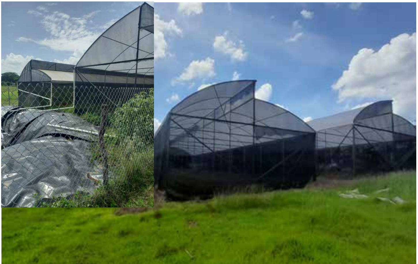
Completed Constructed greenhouses and fenced catchment pond
