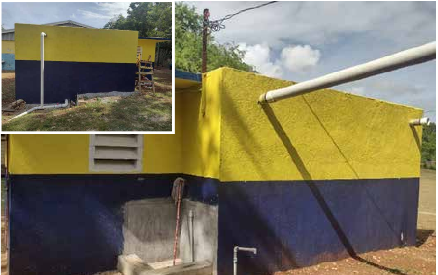
Completed tank with conveyance pipes installed
