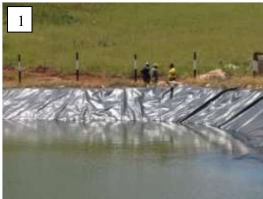
Photos: 1 & 2 - Completed fenced pond with liner at Old England.
