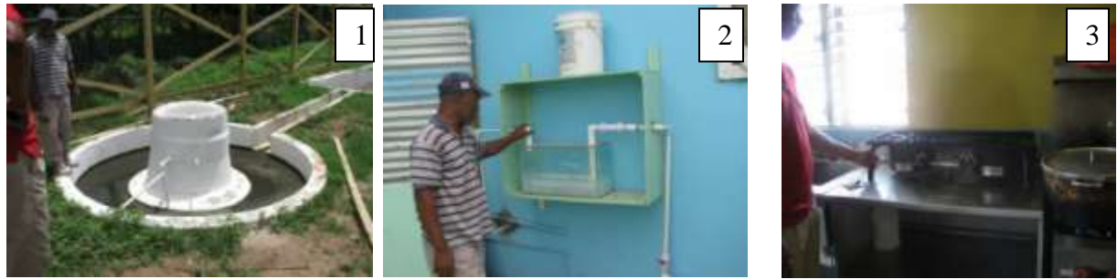
Photo 1: Biodigester chamber at the Sunbeam Children’s Home. Photo 2: Demonstration of biogas system. Photo 3: Biogas being used to generate biofuel in the kitchen at the Children’s Home.
