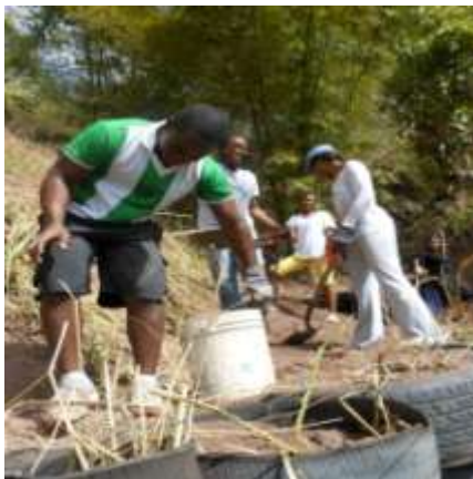
Youths at work constructing retaining wall from used tyres
