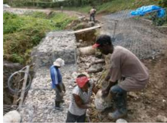
Construction of retaining wall with gabion baskets by the Jeffrey Town Farmers Association in St. Mary, Jamaica
