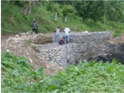
Construction of retaining wall with gabion baskets by the Jeffrey Town Farmers Association in St. Mary, Jamaica
