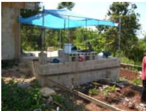
Construction of placement area for water tanks and adjoining abattoir
