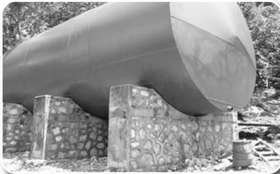
Refurbished Storage Tank at Williamsfield
